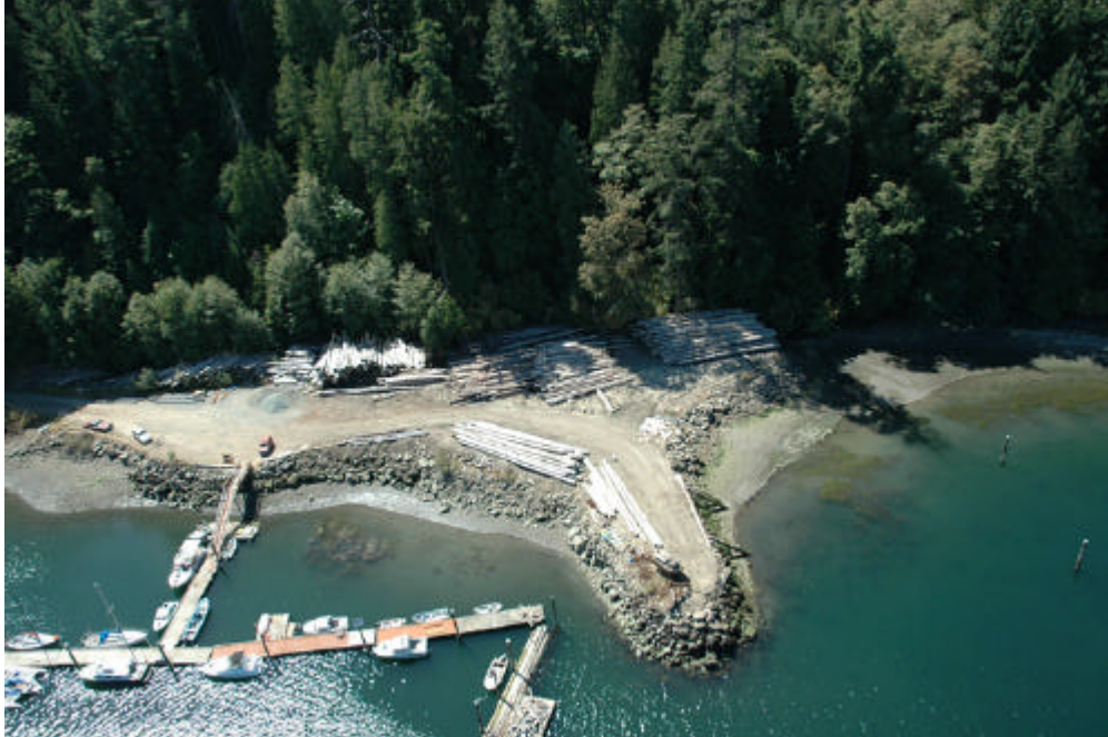
Figure 8 Man-Made Shore Type --Most of the modified shoreline in the Gulf Islands National Park Reserve is rip rap or landfill. This example from Lyall Harbour on Saturna Island is a log load-out site with rip rap, landfill, and wooden docks.
